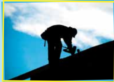
Roofing for staff offices
