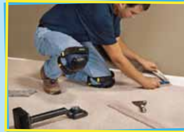
New carpeting in bedrooms and hallways
